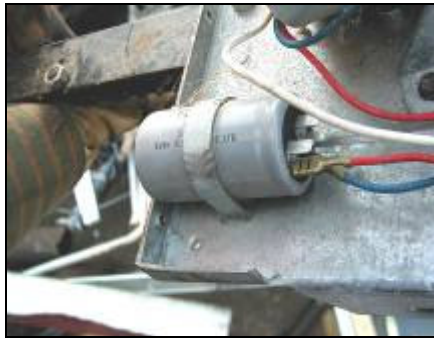
Prohibited: Capacitor in repaired fridge
