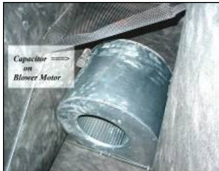
Prohibited: Capacitor on blower fan motor
